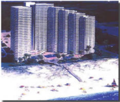
Monte Carlo Condominium - USA
