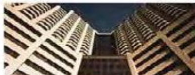
Renaissance Plaza Commercial Office & Residential Complex
