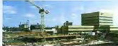
Vallialla Executive Centre - Etobicoke Crang & Boske Architects Inc.
